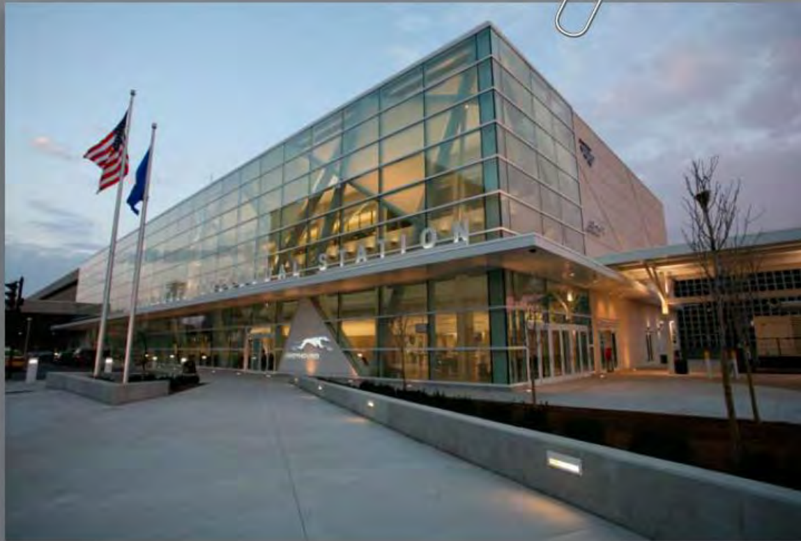
Milwaukee Intermodal Station
